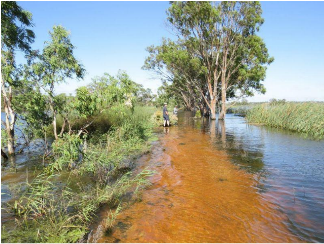
The levee bank got a bit damp. Photo: H. Bean
